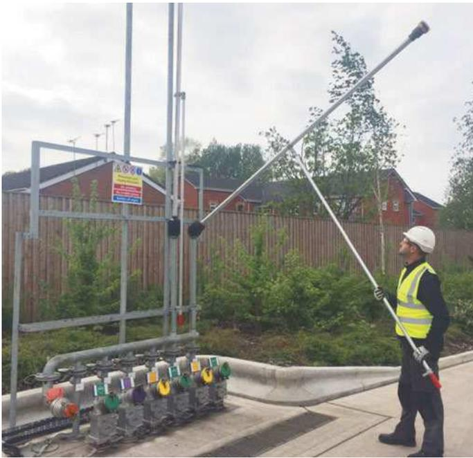
EROS Easy Riser - bringing pre-vac valve maintenance down to earth
